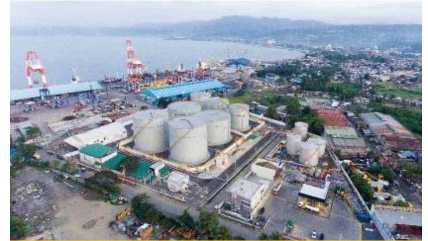
North Mindanao Import Facility
