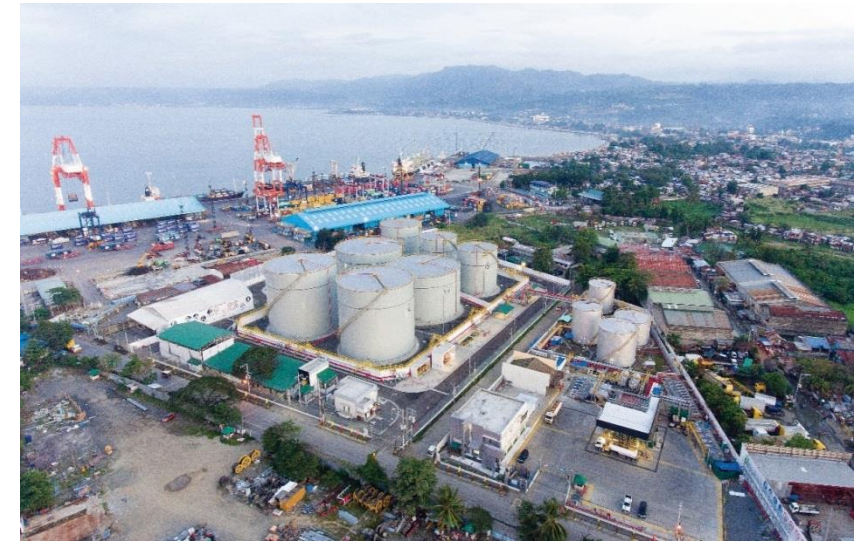
North Mindanao Import Facility
