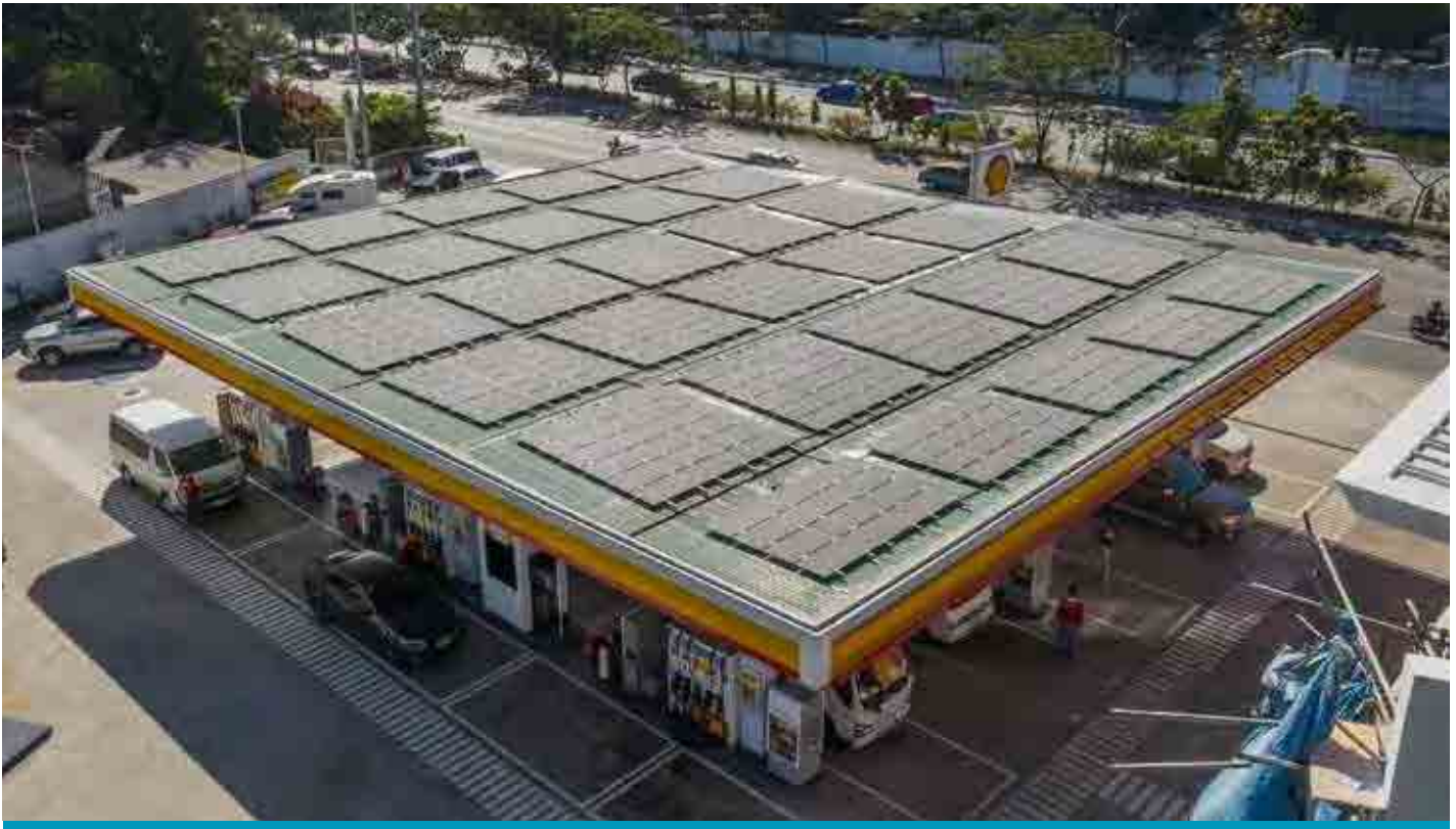
In Picture: Solar panels powering the Shell station
