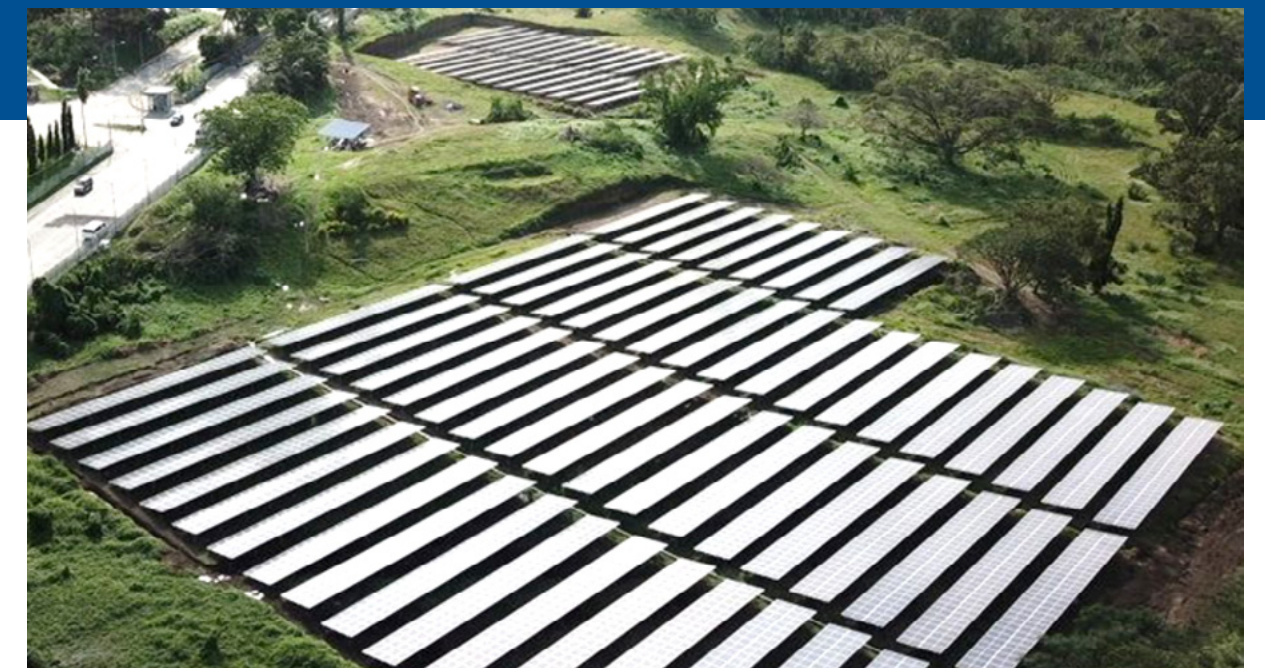
The in-house solar farm, which covers ~15% of power demand of the Terminal, is powered by 5,220 solar panels and seven inverters.
